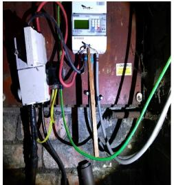
Two examples of electric meters being tampered with and bypassed
