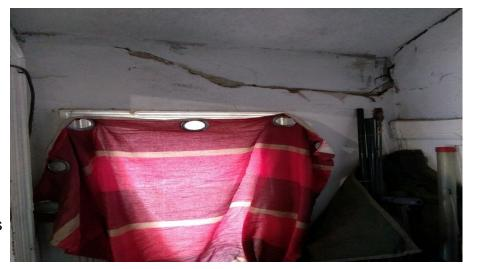
Plaster coming away from lintel above window, caused by missing pointing to the outside and moisture penetrating the brick skin.
