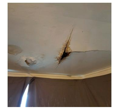
Leaking from the room above, over a period of time, led to the ceiling giving way and collapsing.
